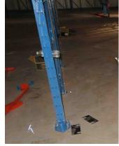
Levelling shims on the floor near metal upright where workers were installing racks.
