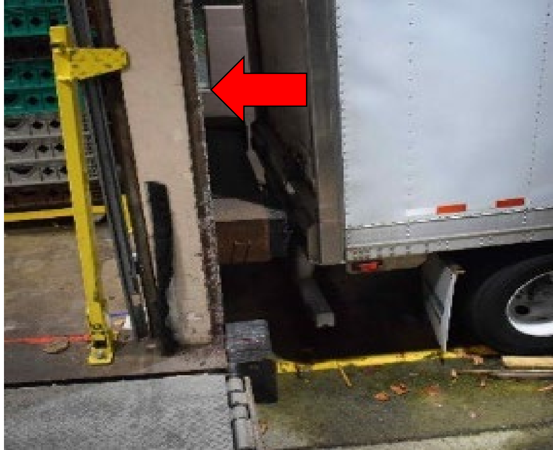
Photo 1. Arrow shows loading dock wall where the clerk was crushed by the trailer.
