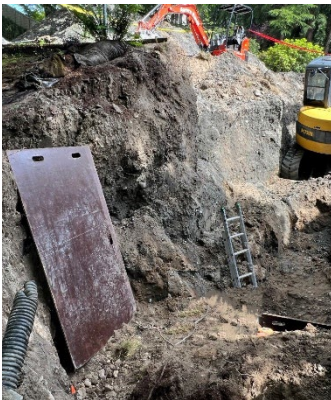
Unbraced steel shoring plate resting against trench wall.
