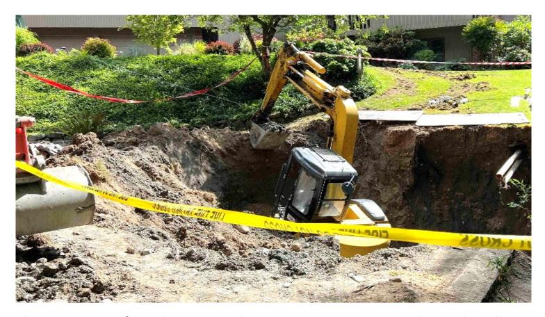
**Photo 1**. View of incident scene showing steep, unprotected trench walls.
