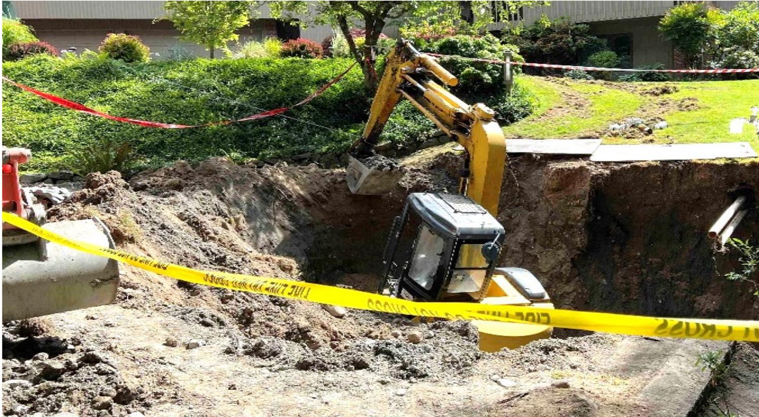
**Photo 1.** View of incident scene showing steep, unprotected trench walls.
