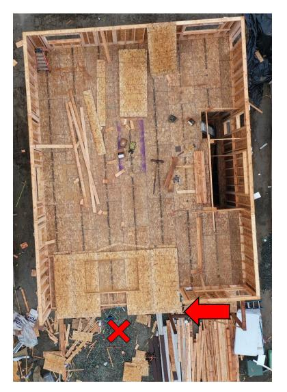
**Photo 3**. Aerial view of upper floor with arrow showing wall sheathing extending over unprotected edge.
