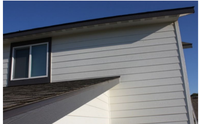
Patio roof (in the lower left of photo) where the installer was standing and prying on the upper roof when he fell.
