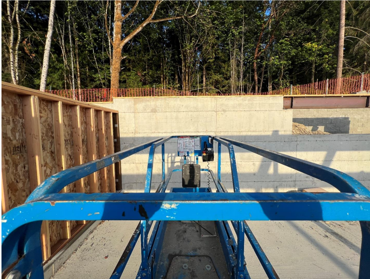
Photo 3. Top guardrail of lift platform.
