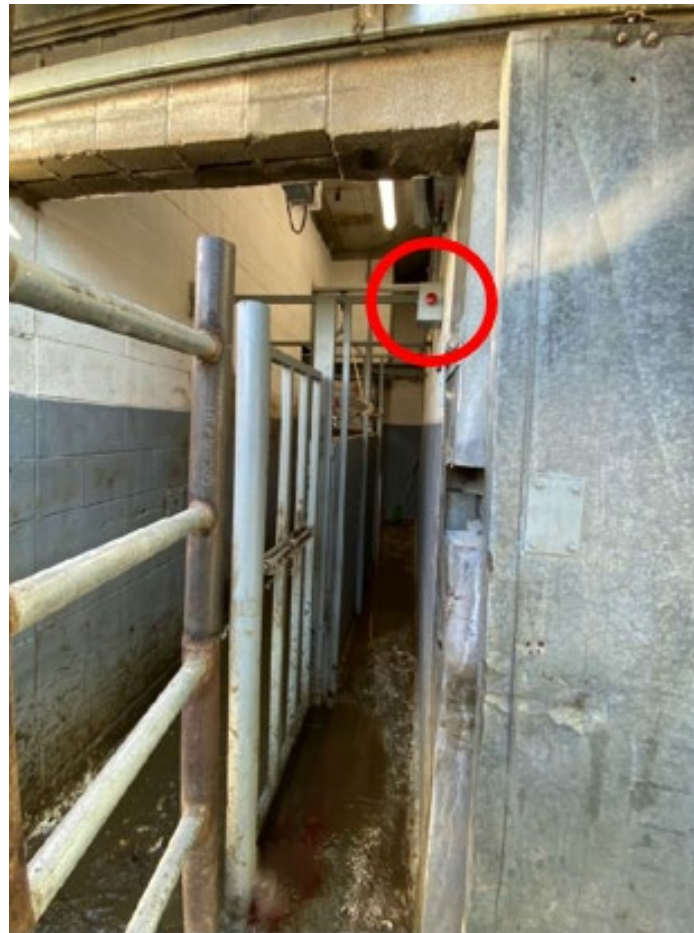
Photo 3. Walkway between barrier on left and door on right. Circle shows inside door activation switch.
