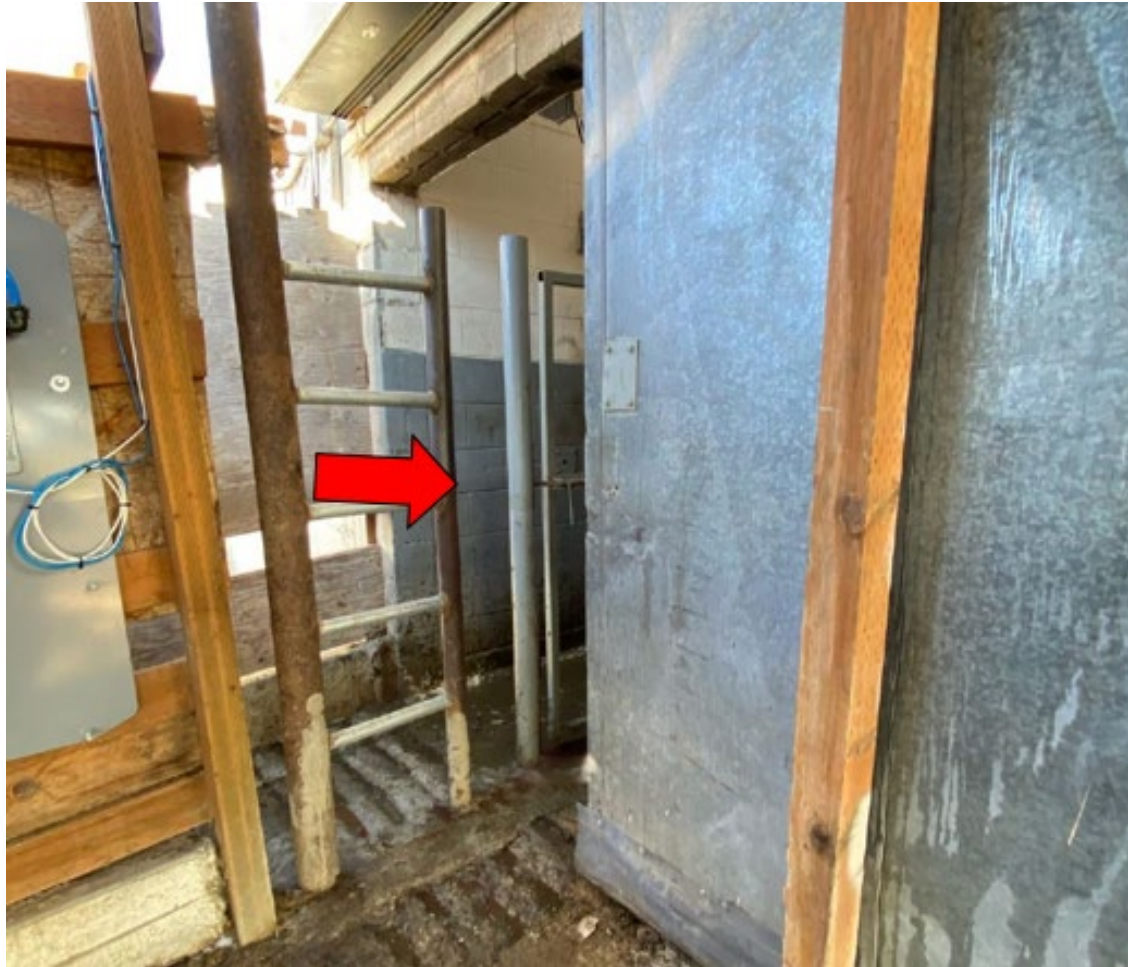
Photo 2. The door opened and closed by sliding through the gap in the barrier.
