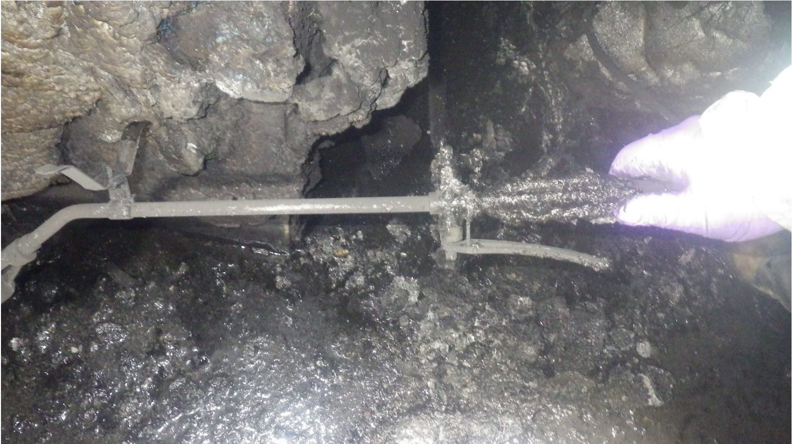
Photo 4. Handheld propane torch used to heat adhesive.
