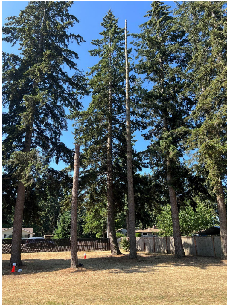
Photo 4. Tree removal job site.
