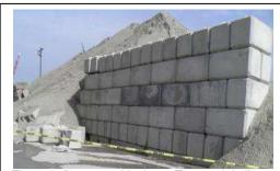
These walls can tumble down. Too much bulk material exerts enough sideways force to cause concrete blocks or whole sections of walls to suddenly collapse.
